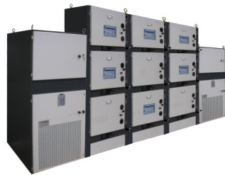
PTM with two transformers, two incoming, one coupling and six network departure
