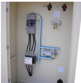
low-voltage compartment
