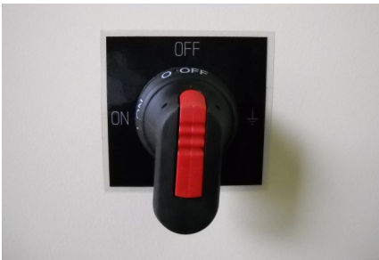
950 V Load break switch
