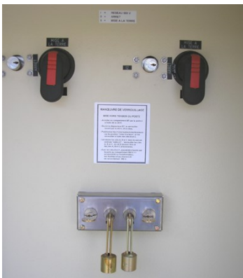
950 V load break switch and lock
