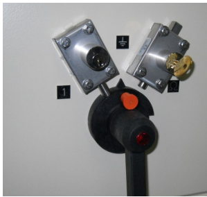
Isolating and earthing switch with lock
