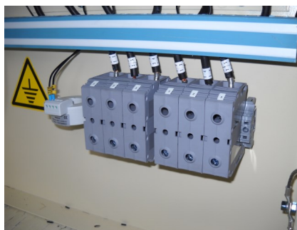
Bornes de Raccordement 950V
