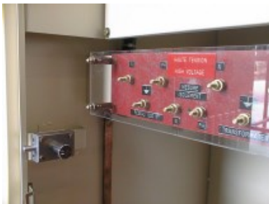
Plaque de Raccordement 3200 V
