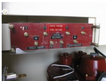
Plaque de Raccordement 3200 V
