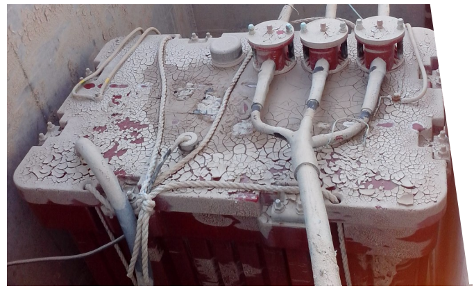
Highway, Middle East, lighting
