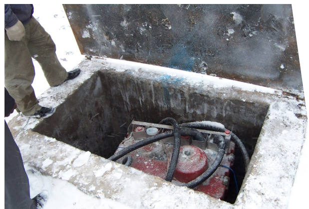
Roads, China, lighting supply
