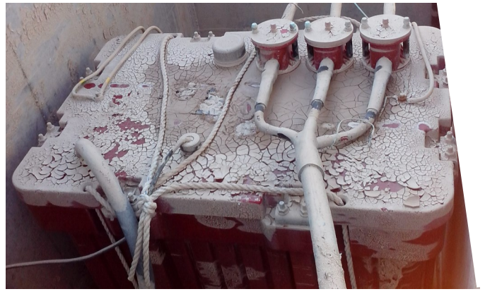
Highway, Middle East, lighting
