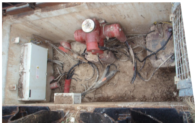
Grands sites, France, éclairage parkings
