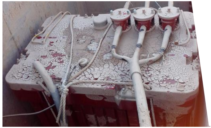
Highway, Middle East, lighting
